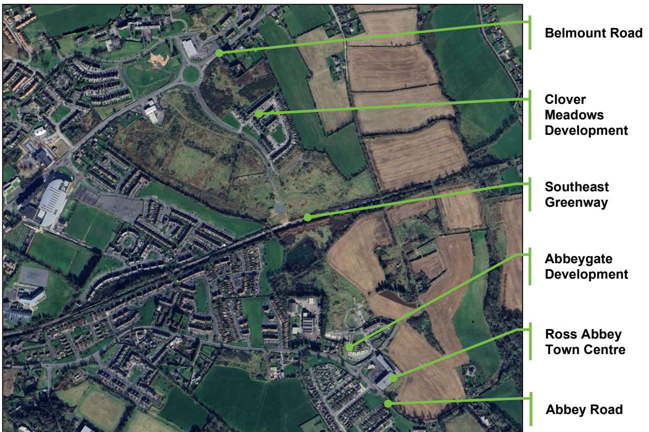
Figure 3-1: Development Site Aerial View
